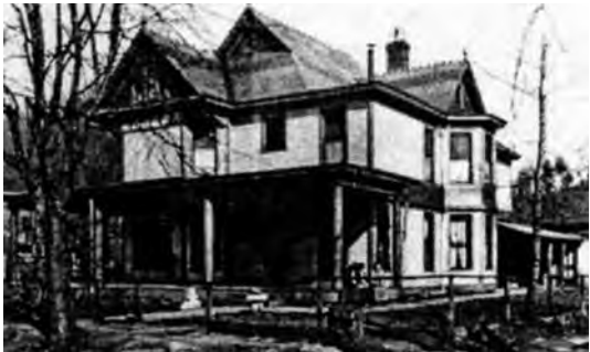
Figure 2.13 Irvinton House, the former US Public Health Service Trachoma Hospital in Pikeville, Kentucky (McMullen J. The government’s work in the eradication of trachoma. Mod Hosp. 1917; 9:163–5, reproduced by Allen & Semba, 2002 (74). Reprinted from Survey of Ophthalmology, 47, Allen SK, Semba RD, The Trachoma “Menace” in the United States, 1897 to 1960, 500–9 © (2002), with permission from Elsevier).
