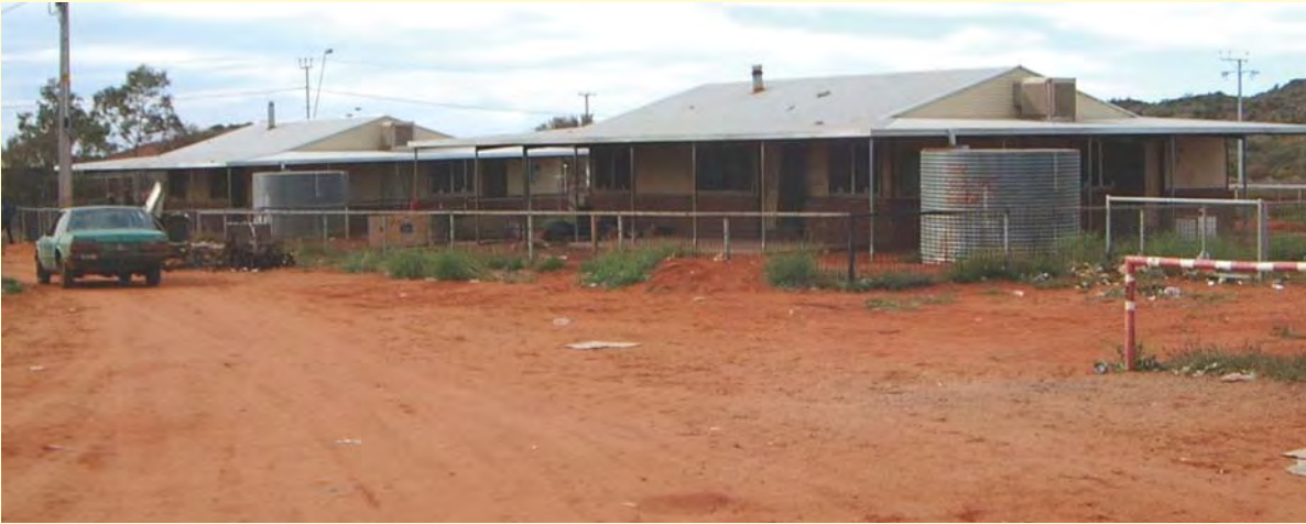
Figure 10.16 Aboriginal housing of reasonable standard in Central Australia. The key to adequate housing is regular and ongoing maintenance and the provision of sufficient houses so that each family has their own functional house.
